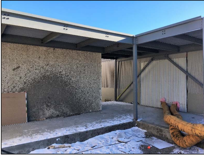
Photo 4: Link to New Modulars Under Construction
