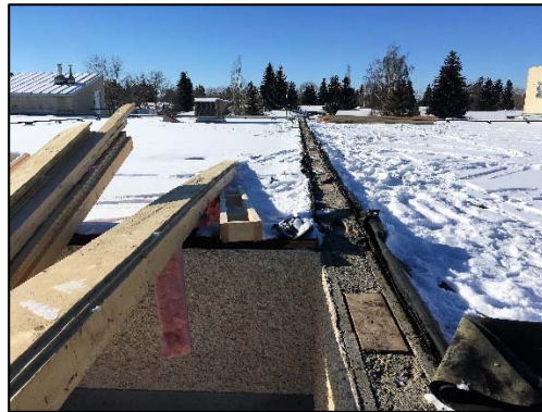
Photo 3: Roof Replacement Underway
