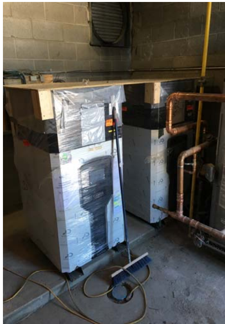
Photo 2: New Boilers Awaiting Installation
