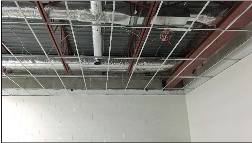
Photo 1: Installation of T-Bar Ceiling in Student Gathering Area
