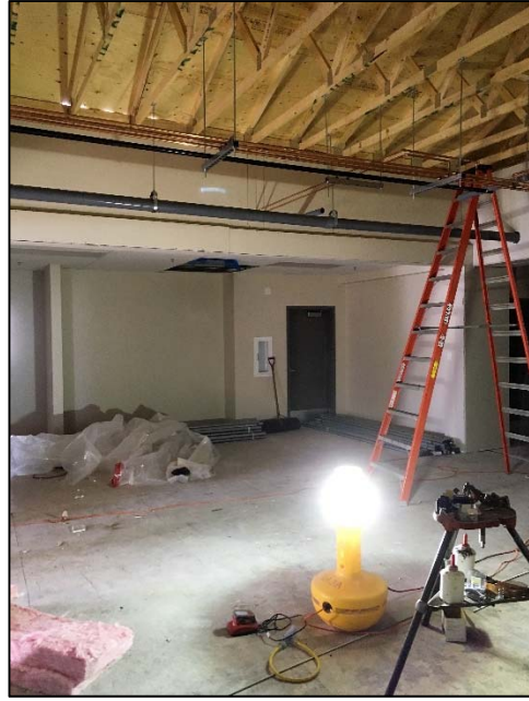
Photo 5: Construction of Breakout Area in New Modular Classrooms
