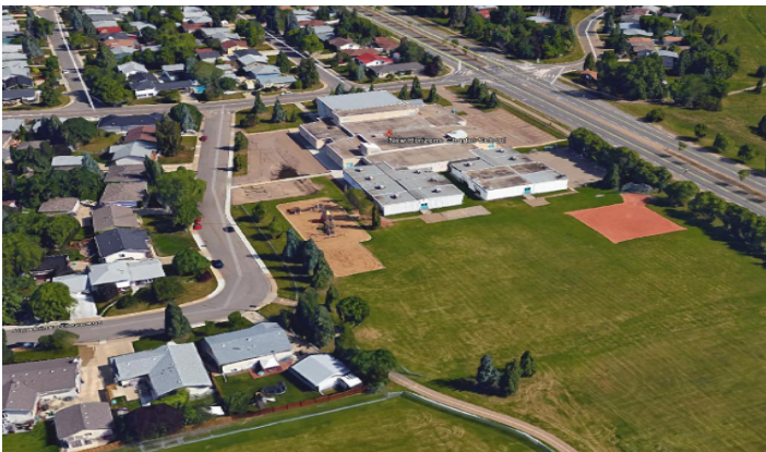
Existing School View
